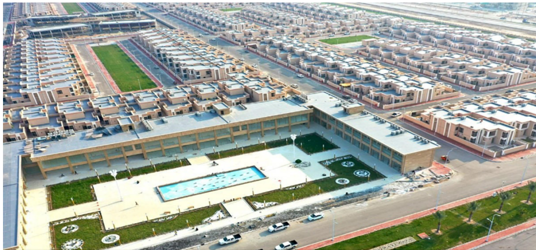
Figure (6). The Horizontal Residential Units of Al Narjis City -Project field visits
