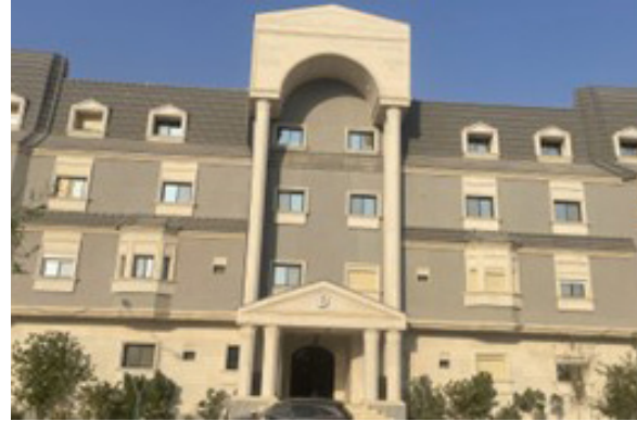
Figure (19). Western patterns in multistory buildings. Source: Author
