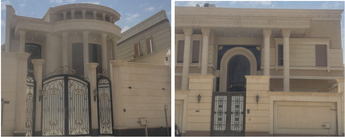
Figure (10). Columns and Fabricated iron gates. Source: Author
