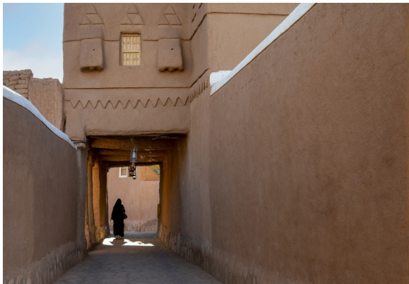
Figure (12). Few openings in the traditional facades (Heritage commission, 2023)
