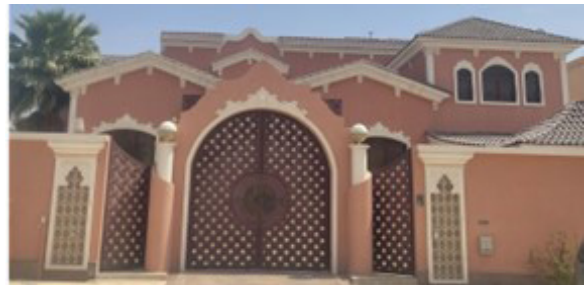
Figure (14). The fences in the modern villas. Source: Author
